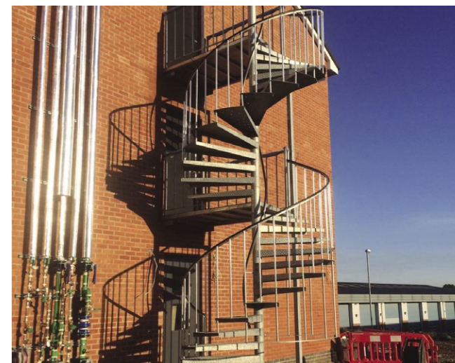
External spiral - Larkhill Contractor/ Aspire Defence
