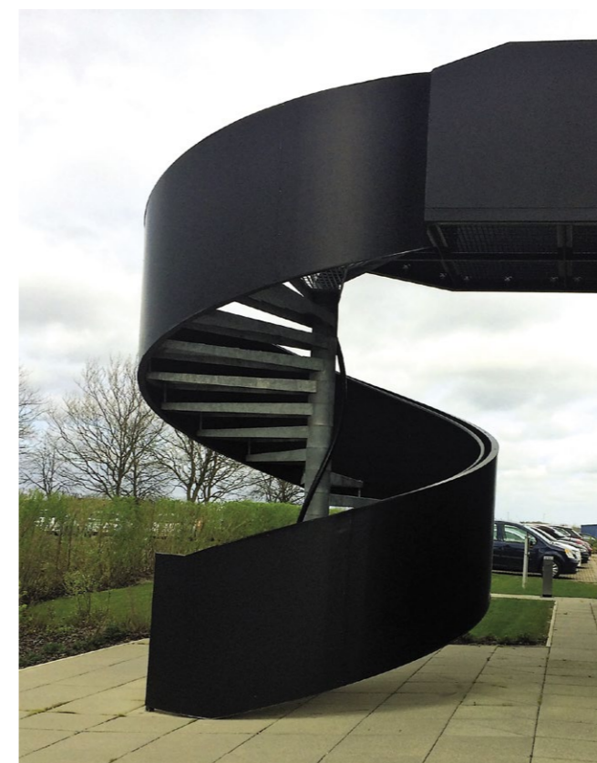
External spiral with full height balustrade - Alconbury Weald Contractor/ Kier Construction
