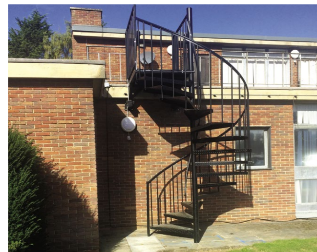
External escape stair - The Leys School, Cambridge Contractor/ TJ Evers
